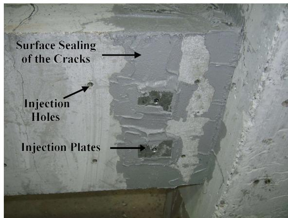
Fig. 2 - Sealing of the exposed surfaces of the cracks and injection plates
