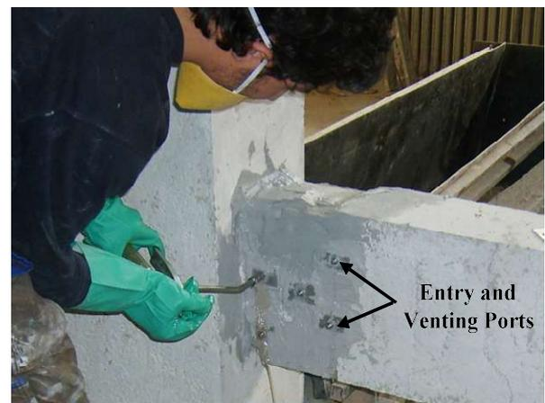
Fig. 3- Epoxy injection
