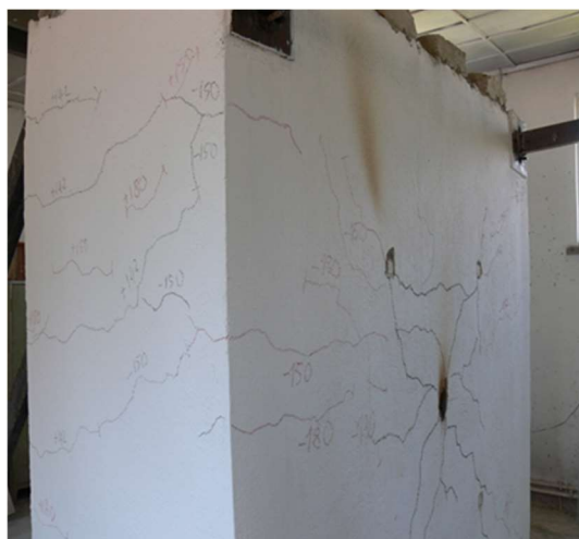
Fig. 7 - Crack pattern of the SMW.
