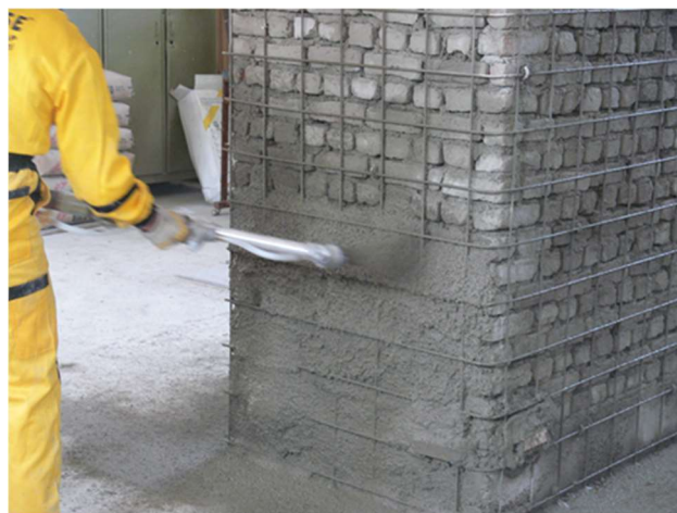
Fig. 3- Spraying concrete on the surface of the wall
