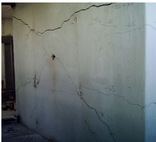
Fig. 6 - Crack pattern of the URM.
