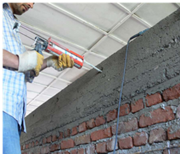
Fig. 2 - a) Mesh of steel beams anchored to the floor anchor with epoxy resin.
