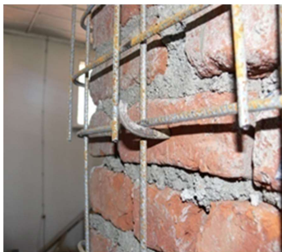
Fig. 2. b) Steel mesh anchor on the wall
