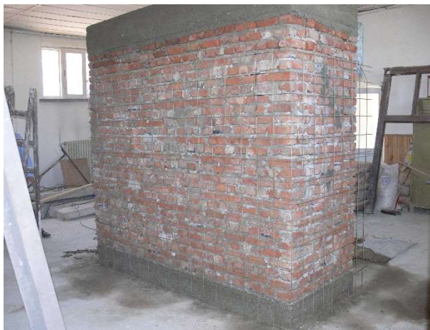
Fig. 1 - Wall coating with steel wire mesh.
