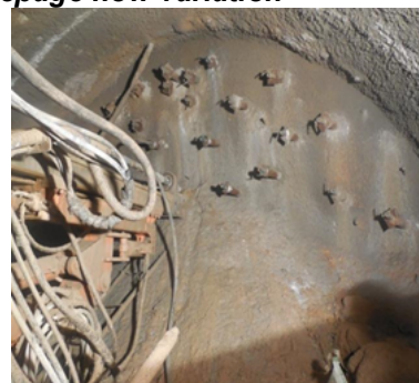
Fig. 7 - Full-section grouting of the face.
