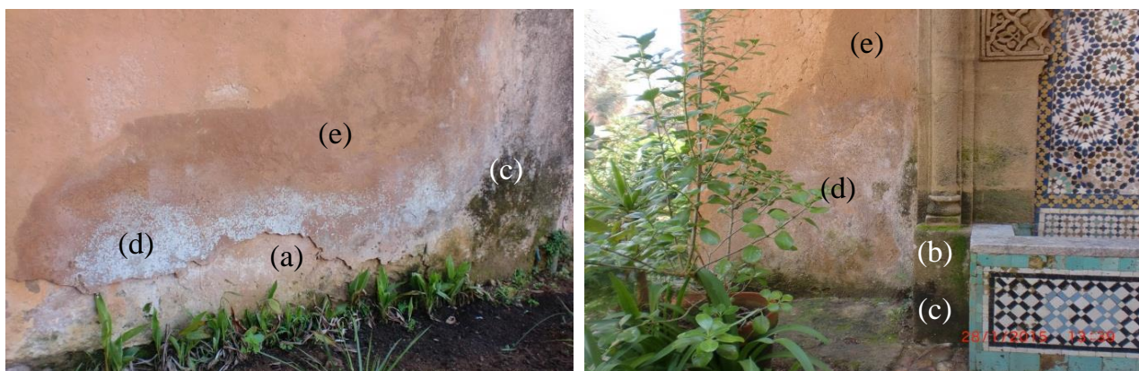
Fig. 2 – Walls bases in calcarenite in the garden of Udayas already restored; soil water rises by capillary transfer in the base, contour scaling initiated on the part in contact with the ground in zone (a) where evaporation is faster than capillary rise, development of green algae (zone b) and lichen (zone c), white efflorescence of salts (zone d) where the water evaporates on the surface, (zone e) always wet.
