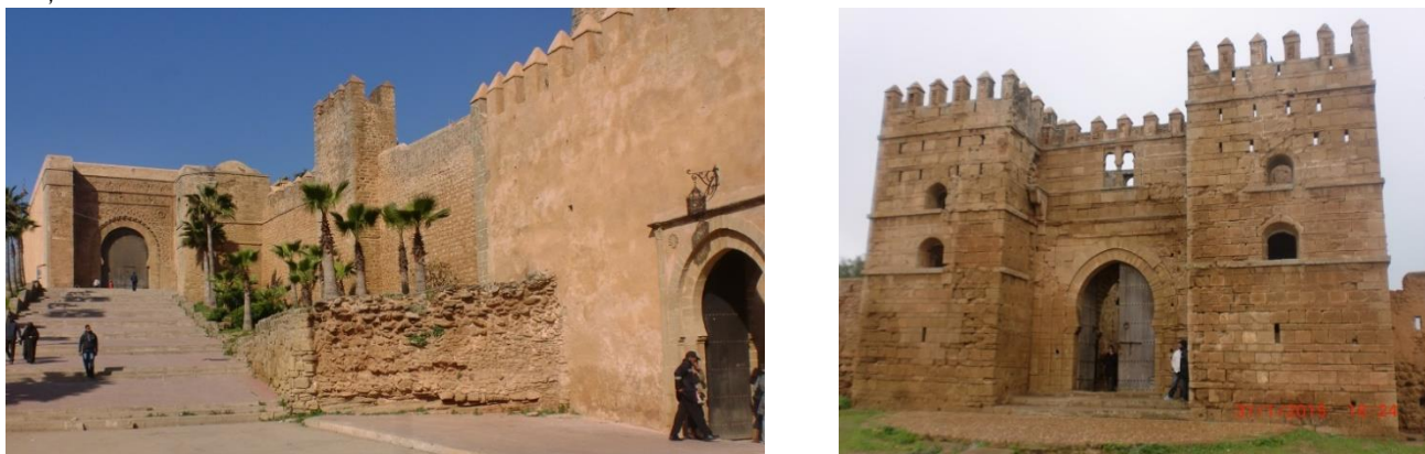
Fig. 1 – Examples of calcarenite historic monuments built in the edge of Atlantic Ocean between Rabat and Kenitra. Left picture: Kasbah of the Udayas located at the mouth of the Bouregreg river in Rabat city. Right picture: Kasbah of Mehdiya situated at the mouth of the Sebou river, about 8 km west of Kenitra city.
