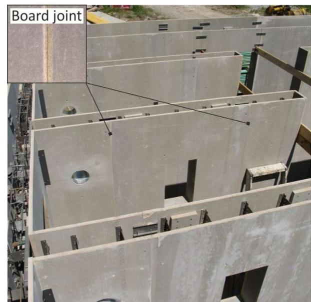
Fig. 6 - Wall formwork elements installed on the construction site with indication of the factory-made board joints.
